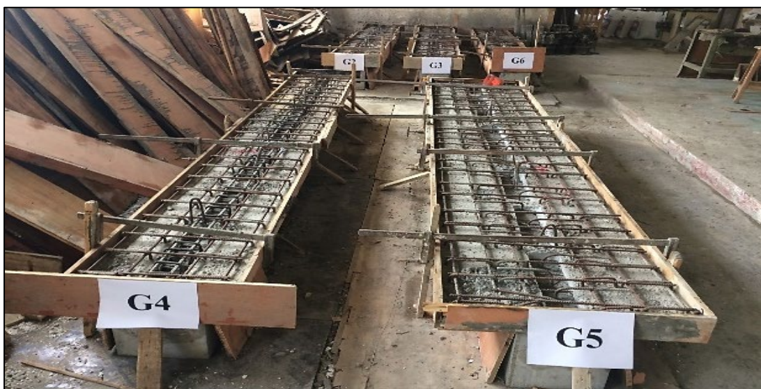
Figure 13: Preparation of casting the rest of topping slab
