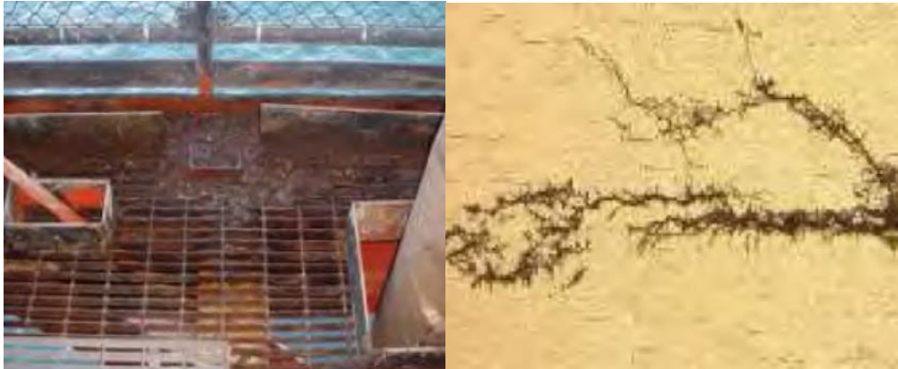
7 8 9 10 11 12 13 14 15 16 17 18 19 20 21 22 Figure 2. Corrosion on gratings and Cracks on plates of Offshore structures [86] 23 24 25 26
