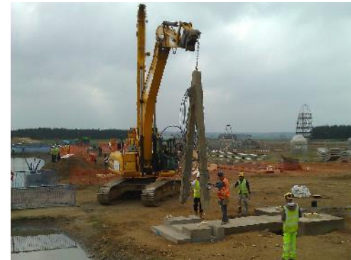
Foundations cast and installing 'A' frame and decks
